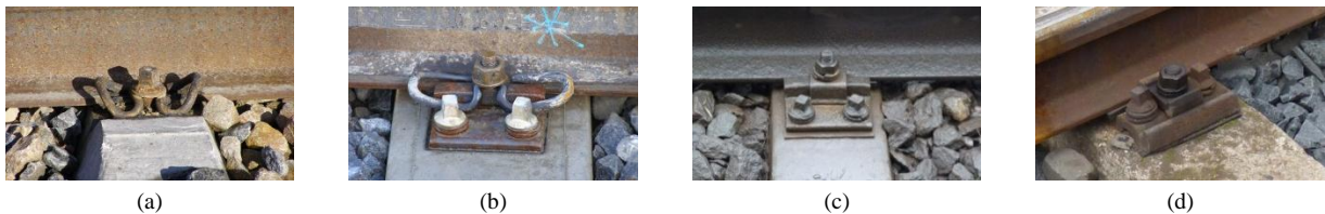
Fig. 2 – Measured construction types of rail fastening systems, (a) direct elastic system W14, (b) indirect elastic system KS, (c) indirect non-elastic system K, (d) indirect non-elastic system with divider heel baseplate [author]
