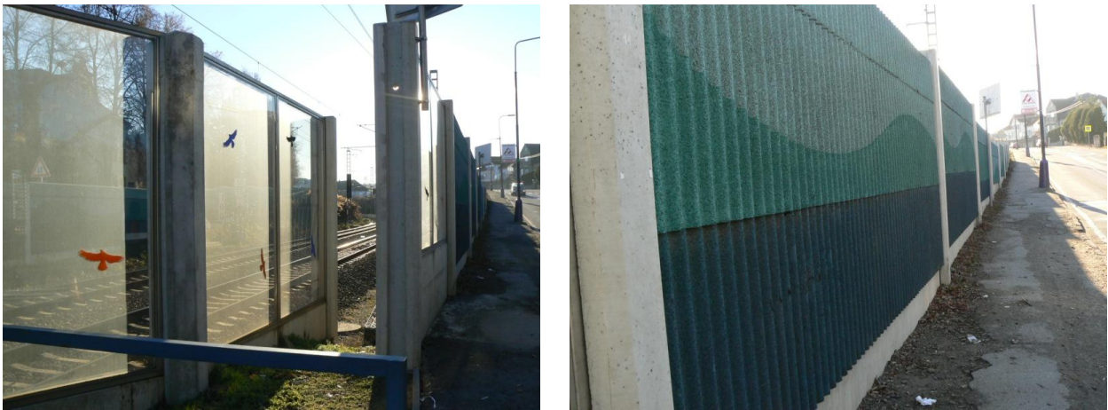
Figure 2,3: Examples of noise barrier in the Czech Republic [author]
